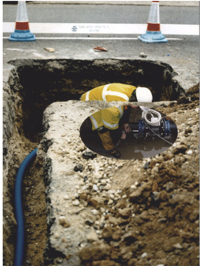
Underground Installation of MagMaster
