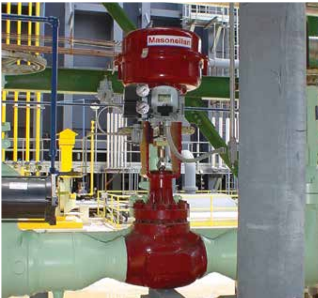
SVI II AP on severe service valve
