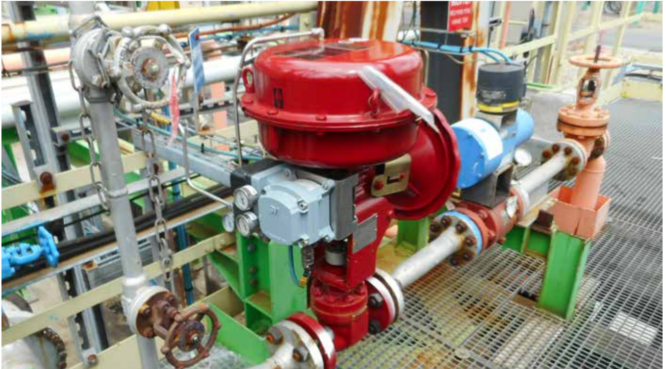
SVI II AP positioner on 21000 Series control valve
